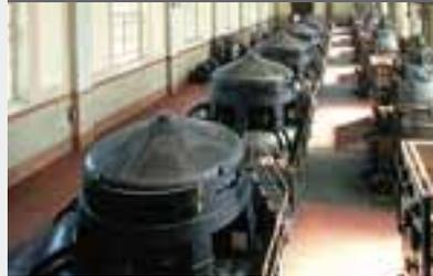
The large drainage plant, with 6 operating pumps, keeps part of the provinces of Bologna and Ferrara free from water.
